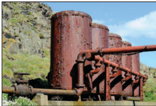
Rusted Compressed Air Tanks
